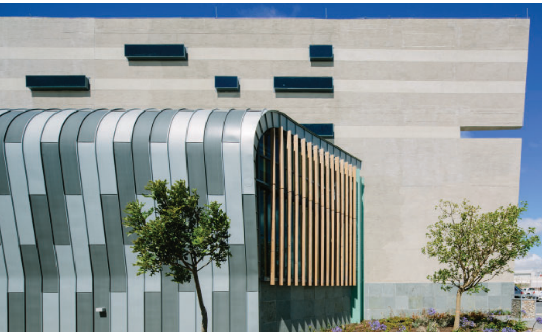
SANRAL Regional Office, Port Elizabeth, South Africa
